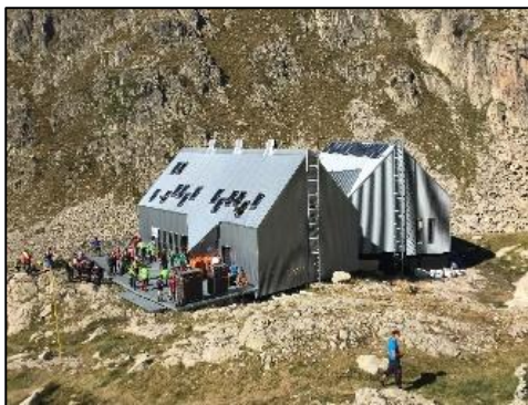
4 kWp of PV
