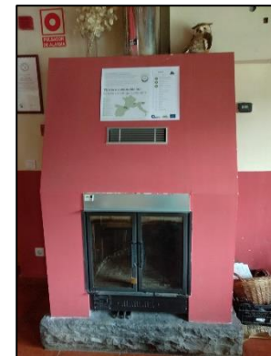
Installation of a thermo-chimney with high efficiency
