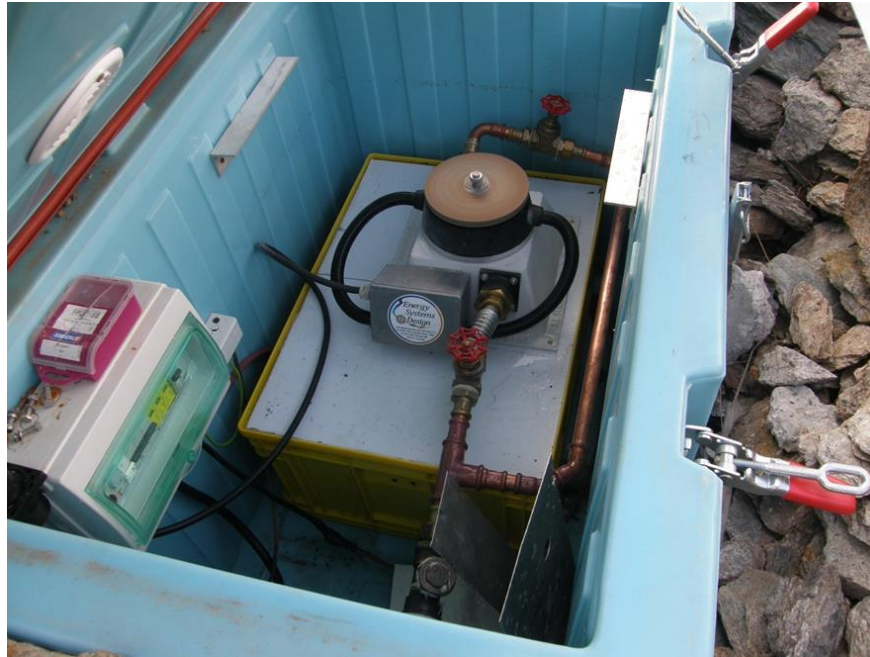
FIGURE 7. DENT PARRACHÉE HYDRO TURBINE (600w)
