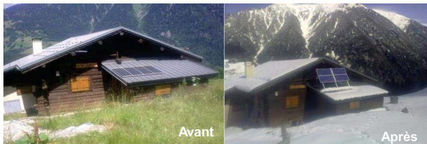
FIGURE 4. PREVENTING SNOW COVER OVER SOLAR PANELS (© COURTESY OF INES)
