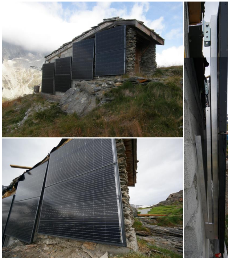
FIGURE 2. VERTICAL PV PANELS INSTALLATION
